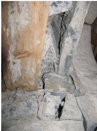
Damage above a "closed" window opening
