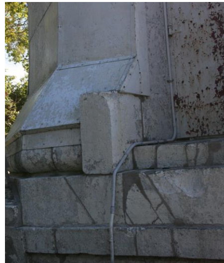
Damaged foundation of lighthouse
