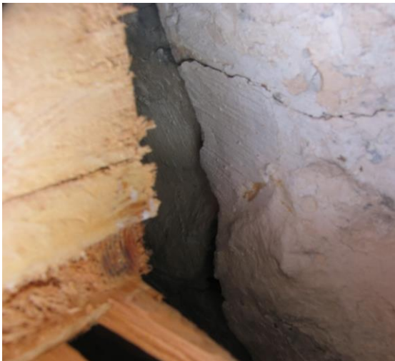
Serious cracking inside Near window opening
