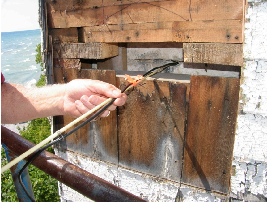
Fig.11: Borescope probing at revealed mortar joint. Quoin masonry appears regular.
