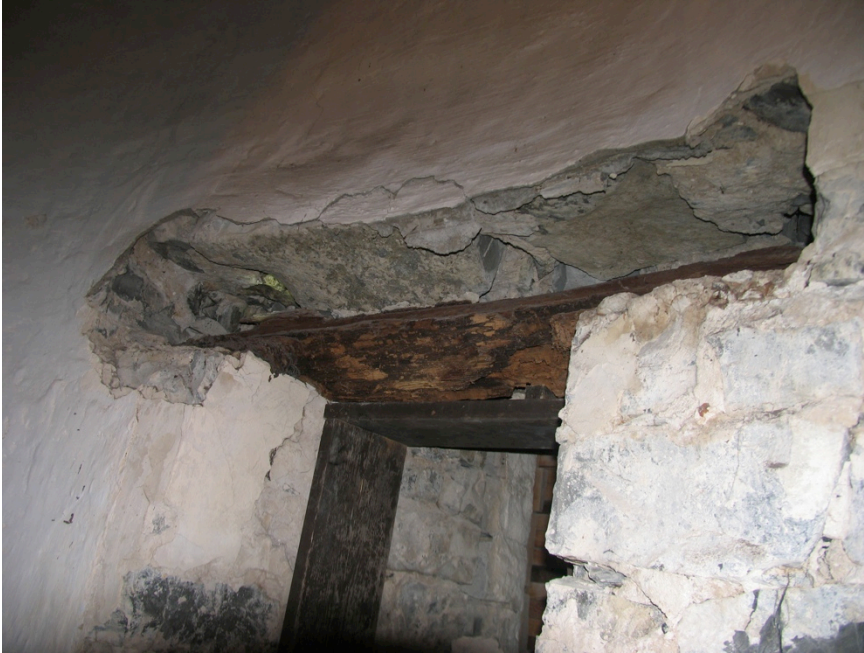
Fig.9: Decayed timber lintel at lowered openings - 2 nd floor
