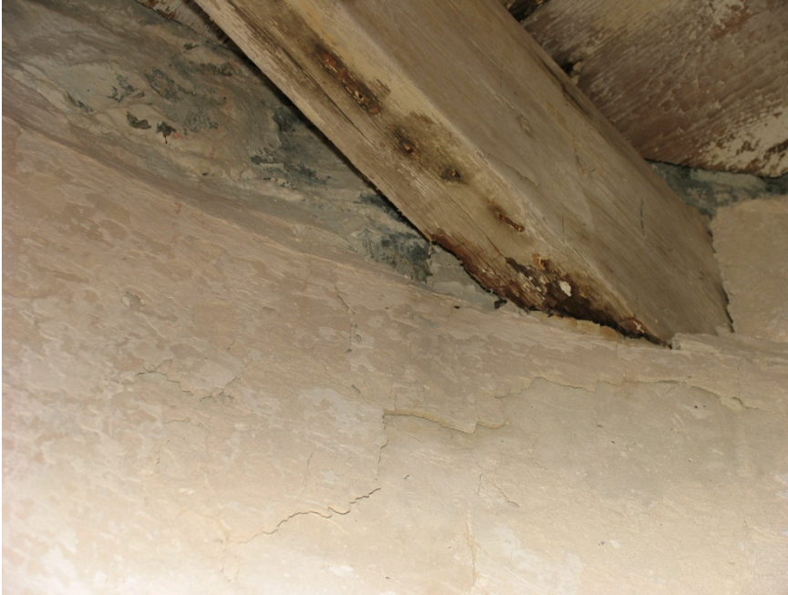
Fig.7: Note decay extending from bearing point at wall. Also lathing? nails
