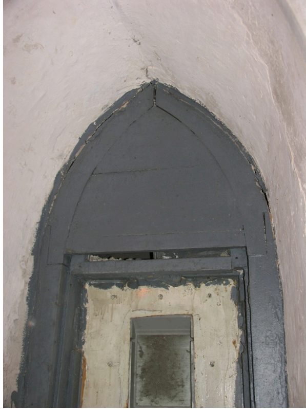
Fig.8: Interior treatment at west elevation. Note surviving upper sash.
