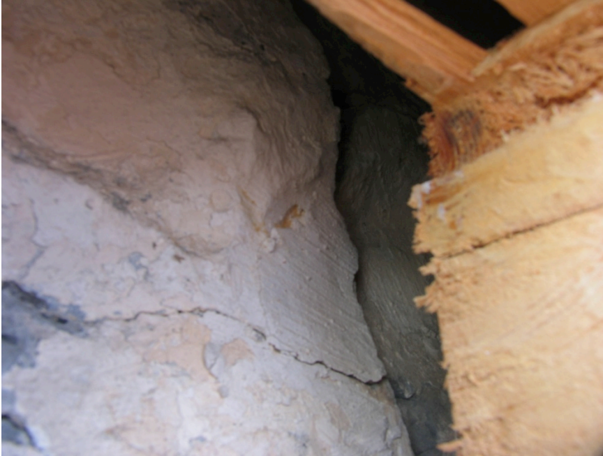
Fig.12: Serious vertical crack and displacement extending from lancet top
