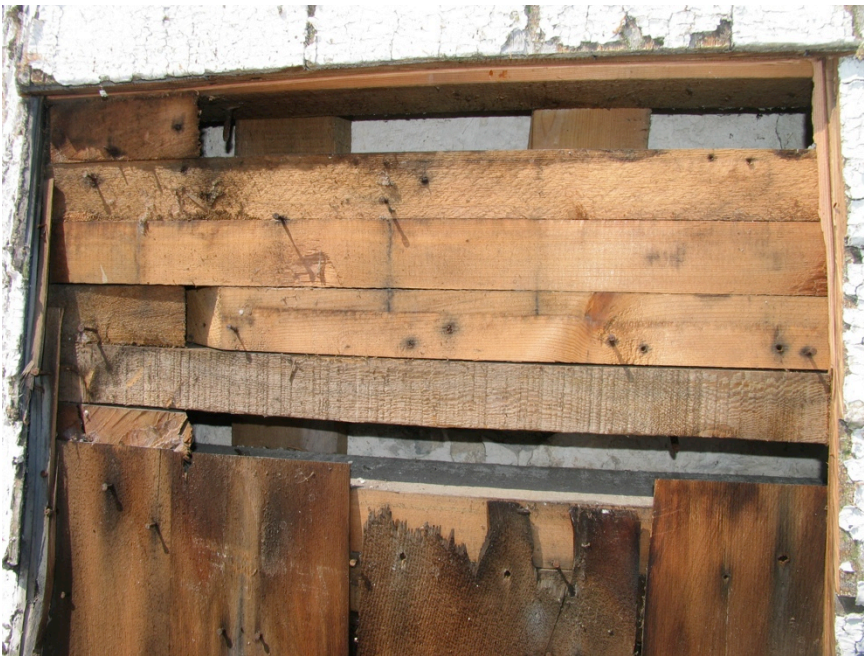
Fig.13: Various girt configurations are used with cross-lapped corbers
