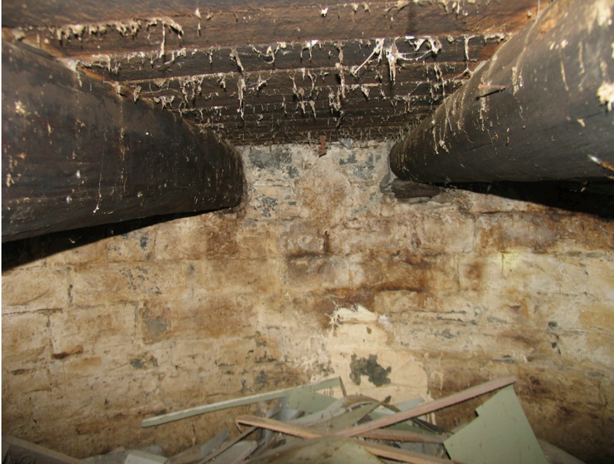
Fig.10: Note creosoted ¾ round timbers and quality of stone coursing
